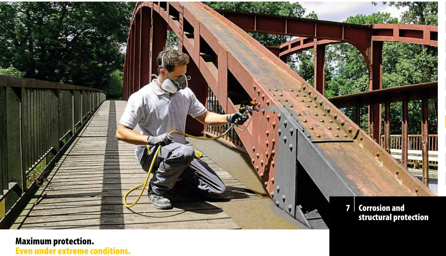
The effects of weather, UV rays, salty air, temperature fluctuations, acids and aggressive substances: the list of influences that can attack surfaces is a long one. Structures used for power generation and distribution, industrial buildings and infrastructure projects are particularly badly affected. Consequent maintenance work in the form of regular protective coatings is essential. WAGNER offers the perfect hardware solutions for especially tough, uneven surfaces.
